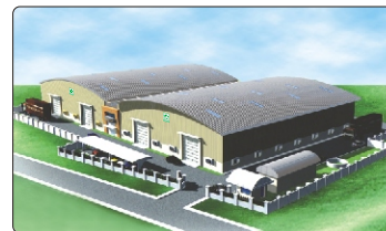
VANJAX FACTORY UNIT -2 (VXC-2)
